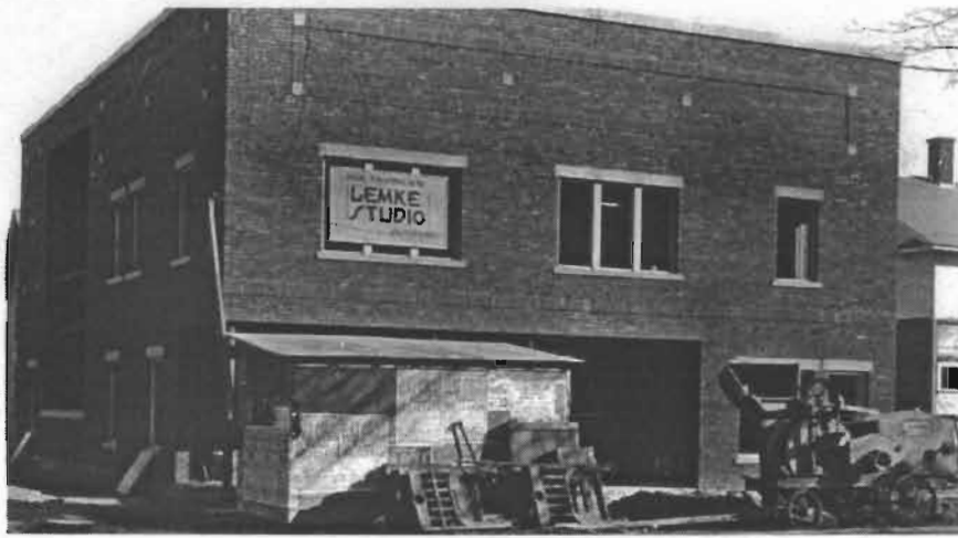
The new Lemke Studio under construction.
